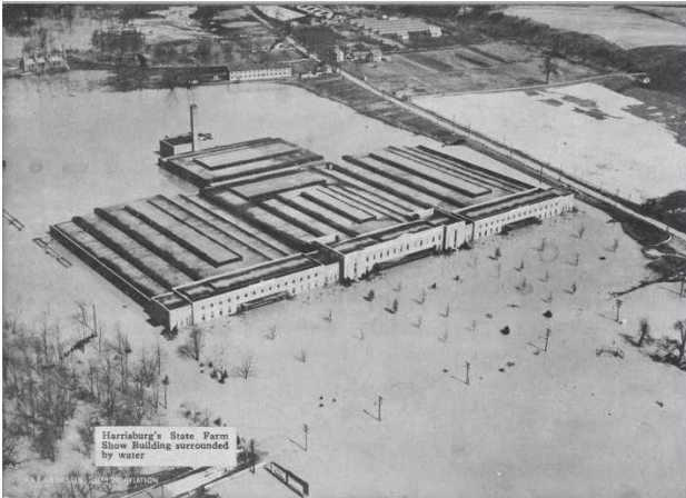
Farm show building during flood of 1936
